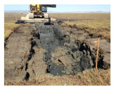
Figure 7. Hanford excavated the southern end of the main channel alignment with an approximately 16ft top width and 5ft depth. The channel top width gradually widens as the channel nears Sonoma Creek to 50 ft top width and 7.5ft depth from marsh elevation. Because of difficult construction conditions and substrate consistency, the side slopes were modified from a 1:1 to a 3:1 slope ratio to ensure channel banks do not slump more than expected.
