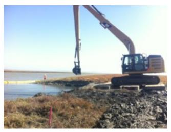
Figure 10. At its widest point, the channel mouth connection point at Sonoma Creek, the channel alignment reaches over 50ft top width and is 7-7.5 ft deeper than marsh elevation.
