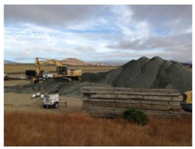
Figure 4. Over 14,000 tons of drain rock was brought into the staging area by Hanford for construction of the permeable "floating" road that is used to access and excavate the channel alignment.
