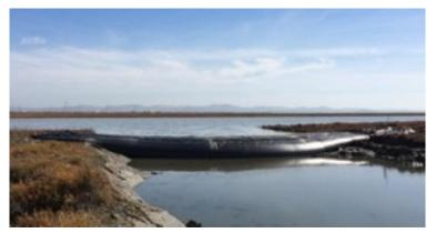
Figure 11. This Aquadam was installed by Hanford A.R.C. as a secondary precaution beyond the placement of the turbidity curtain. This dam moved with the tides but maintained a constant seal at the channel mouth to trap suspended sediment and inhibit access of fish and marine mammals into the construction zone from Sonoma Creek.
