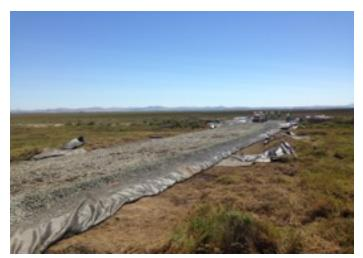
Figure 6. Once the access road was laid, Hanford continued the road south towards the endpoint of the main channel. When completed, the access road to and along the main channel alignment reached just under 1 mile in length.
